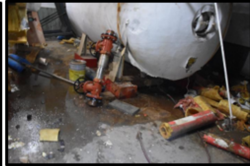
Photos of suppression piping that has been cut out of the system. This is a recent development. These photos were from 3/9/2026, and the pipe had not been like this in previous administrative warrants.
