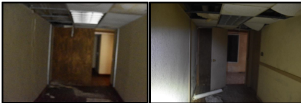
These are photos of doors and walls added to the hallway
