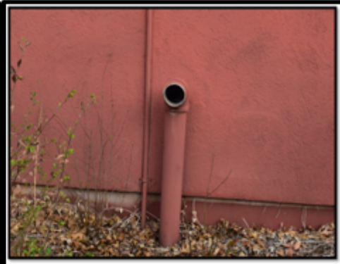
Fire Department Connections removed March 2026
