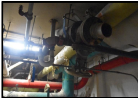
Photos of suppression piping that has been cut out of the system. This is a recent development. These photos were from 3/9/2026, and the pipe had not been like this in previous administrative warrants.
