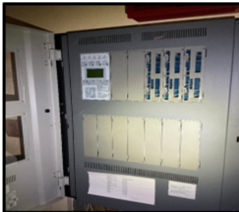
Alarm system – no power, inoperable, no tag
